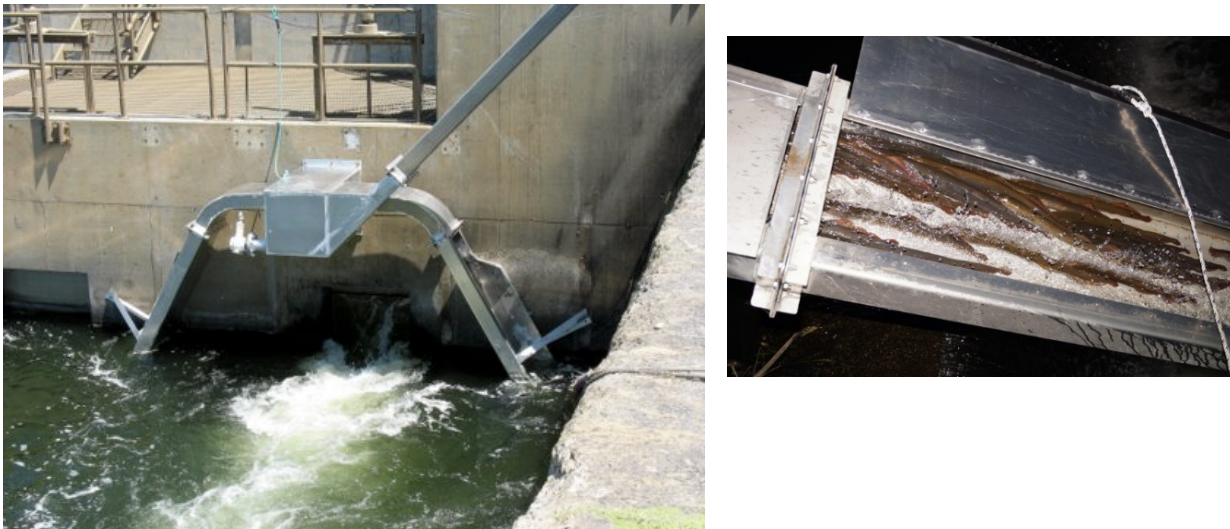
Figure 1. Photos of Three Mile Falls LPS with dual 60° entrance collector ramps that terminate in a large rest box (left). The 45° climbing ramp from the rest box to the exit slide was covered to protect lamprey from predators and reduce algal growth on the ramp (right). This ramp terminated in a horizontal section leading lamprey through an HDX-PIT antenna, into an upwelling box, and down an exit slide to an open trap box in the dam forebay.
