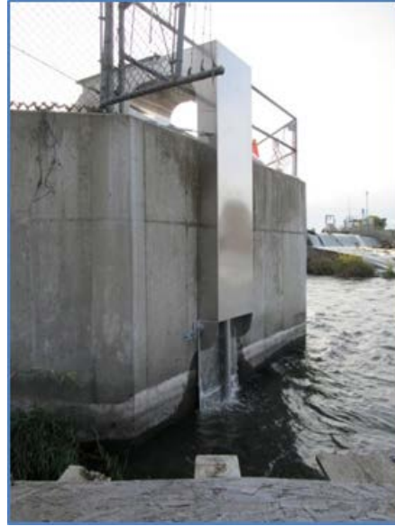
Photo 1. Vertical Wetted Wall Lamprey Passage Structures installed at Prosser Dam (left - Lower Structure, right - Upper Structure). The vertical center guide pipe allows lamprey that are passing along the ladder wall from either directions to sense the flowing water.
