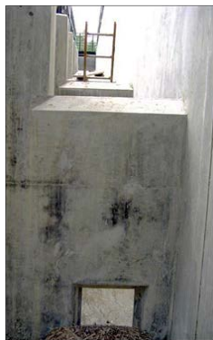
Figure 1. Photos of Pacific Lamprey passage design elements of the River Mill fish ladder. Rounded entrance and filled entrance gate bulkhead slot (left), chamfered orifice and weir (middle) and rounded ladder corner (right).
