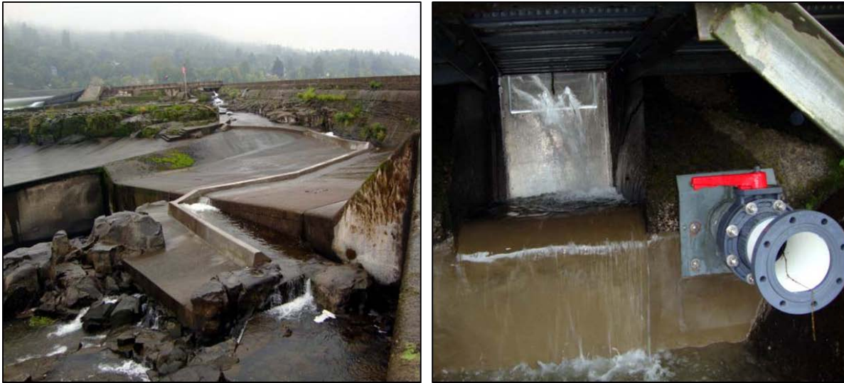
Figure 1. Photos of lamprey curb with flow line open (left) and lamprey exit gate, smooth concrete step, and 8" flow line (right).
